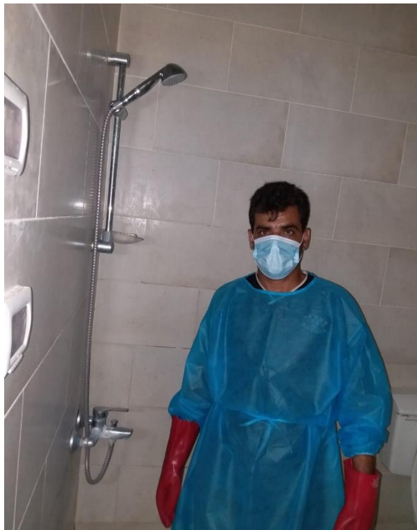
Shower for workers at the end of the working day, all cleaning materials are provided also
