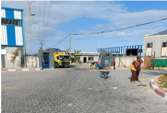
Cleaning of the transfer station entrance
