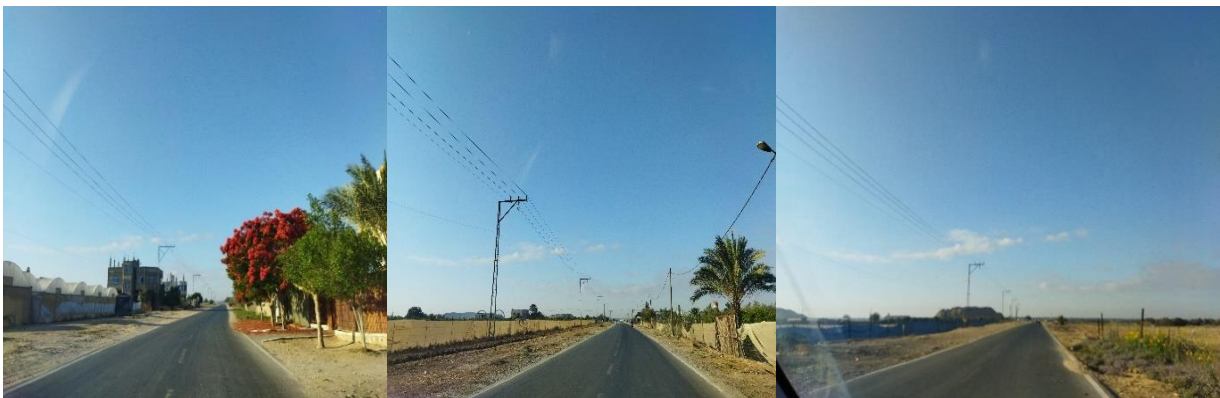
Photo: Sofa Landfill Access Road
