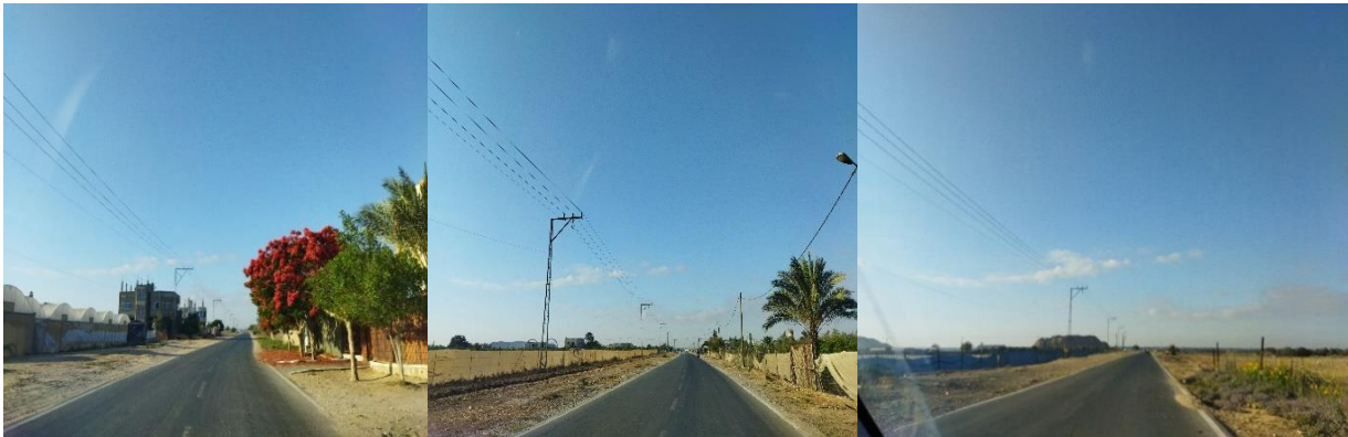
Photo: Sofa Landfill Access Road
