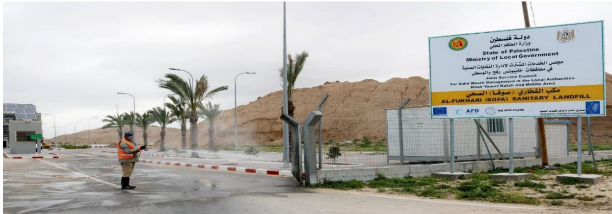
Figure5 . Sterilization of internal roads and facilities landfill
