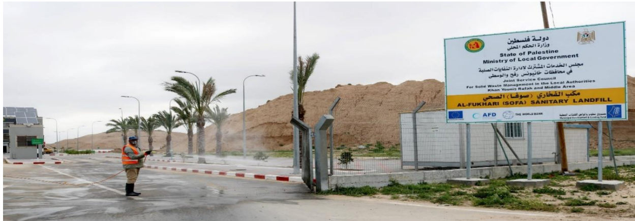
Figure5 . Sterilization of internal roads and facilities landfill
